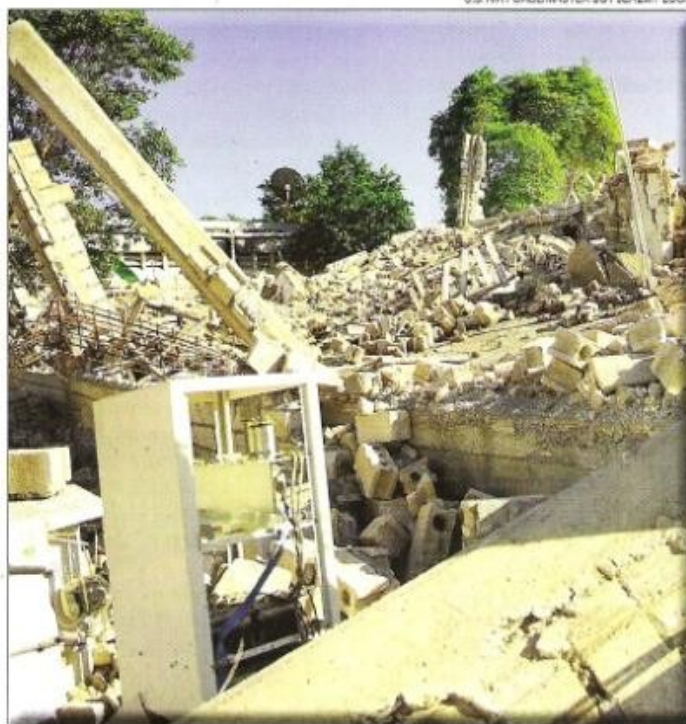
Shown here are destroyed buildings in Jacmel, Haiti. According to local officials about 350 people lost their lives in Jacmel due to the earthquake that hit the region January 12, 2010.
